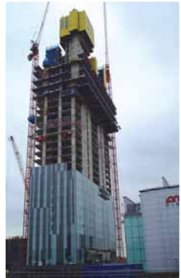
Figure 3: Level 26 with 4m cantilever from Level 23.
