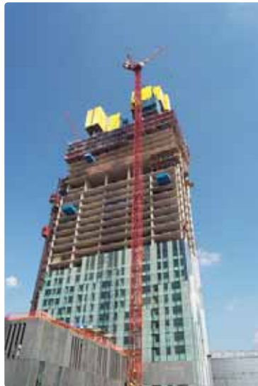
Figure 1: Level 31 crane height 150m.
