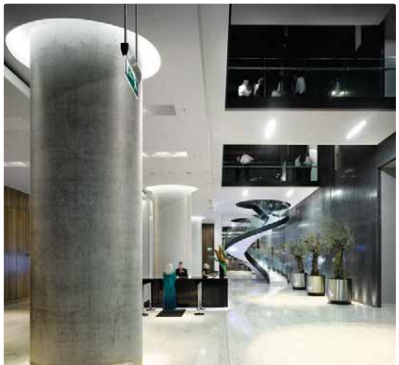
Figure 8 below: Exposed elliptical columns.
