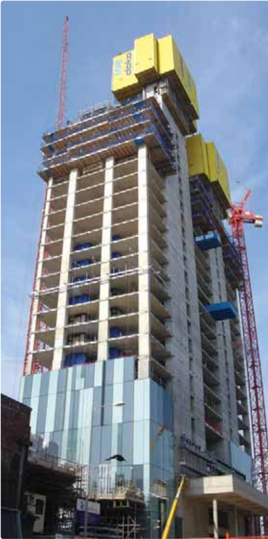
Figure 5 above: Level 21 and Level 3 external swimming pool structure.
