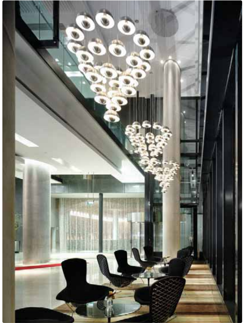
Figure 6 above: 11m in-situ elliptical concrete columns in the Reception.
